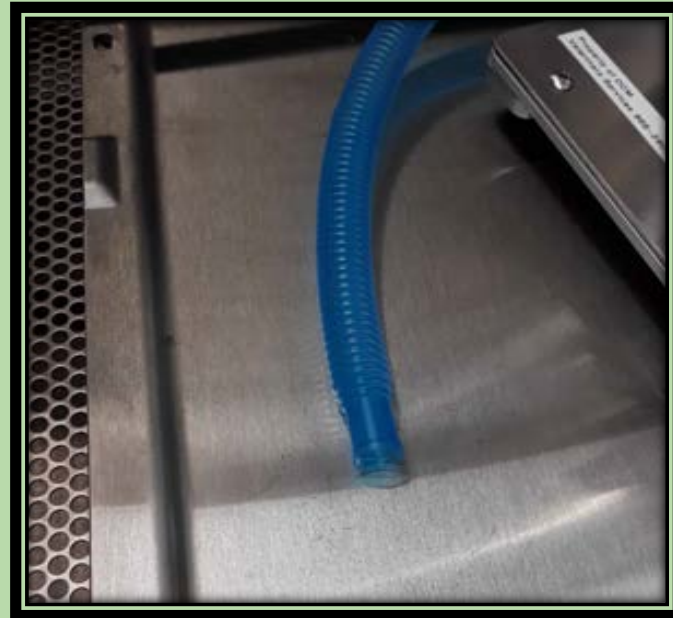
End of exhaust tubing inside ventilated hood
